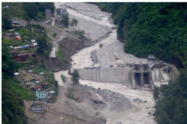
Emergency hazards alleviation in Koshi river
